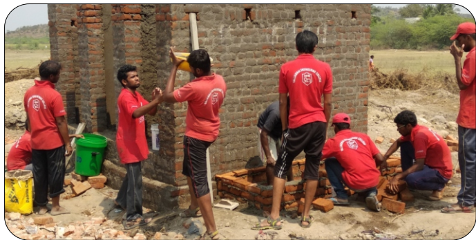
Construction of communal toilets and a soak pit by NSS Volunteers
